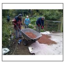
We were tasked with widening the path by the side gate at Withymead.. This involved scraping away the turf and weeds then lining up border boarding before pouring and spreading scalpings over an old carpet membrane.
