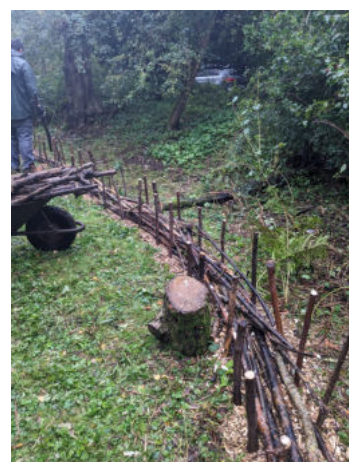
Right: The space between the stakes was then filled with brash (larger material at the base).
